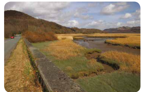
Saltmarshes on the Mawddach Estuary providing key protection to the A496 © Rhoda Ballinger
