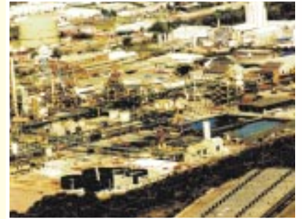
The waste water treatment plant under construction
