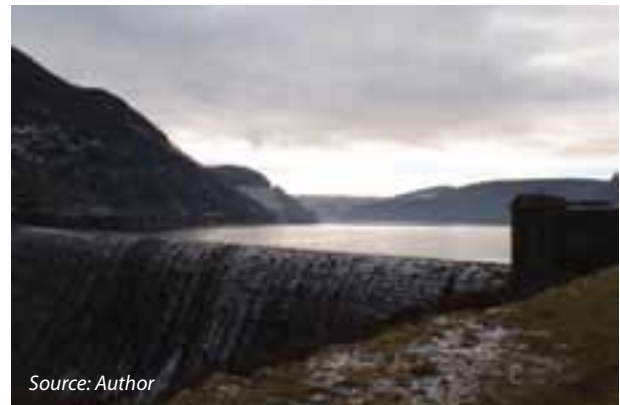
Figure 14. Reservoir owned by Welsh Water Dŵr Cymru, Elan Valley, Mid Wales.
