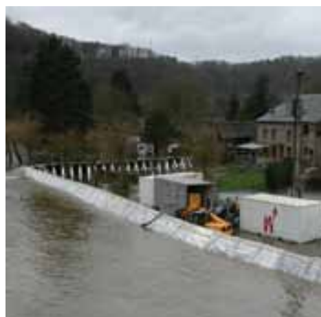
Figure 26. Flood barrier in use, protecting a communication mast and house
