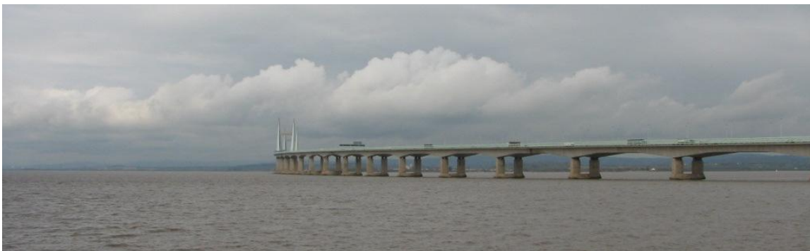
Figure 1: Second Severn Crossing, © SEP
