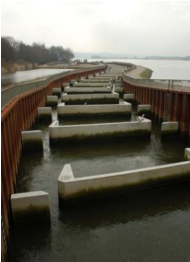
Deep vertical slot Pass
