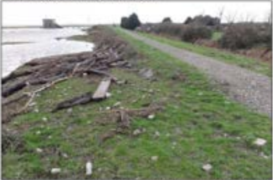
Photo 1: Rhymney wharf flood embankment post 3 January 2014 tidal event (8.03m above Ordnance Datum at Newport 2 gauge)
