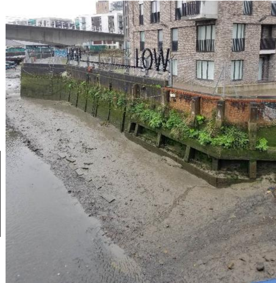
Post-restoration: vertical wall with bolt-on timbers
