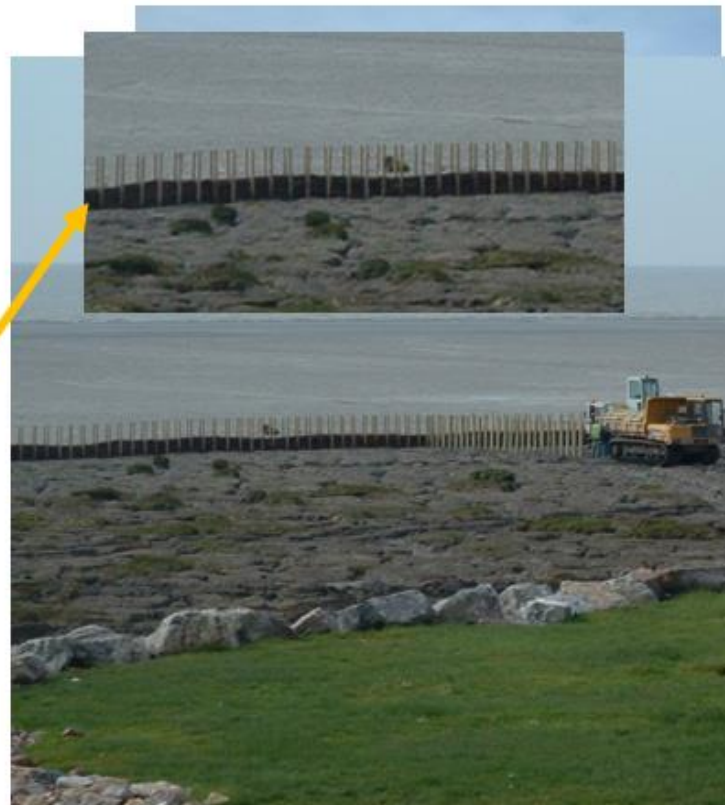
Figure 5.9: Basic setup of a single sedimentation field (also referred to as sedimentation polder) consisting of brushwood groynes inserted in the mudflat to form an enclosure with a tidal inlet (adapted from Colenutt, 2001).
